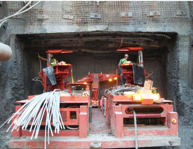
Roof Bolting at White Oak
