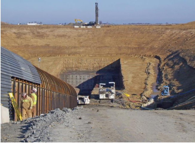
Lively Grove Tunnel
