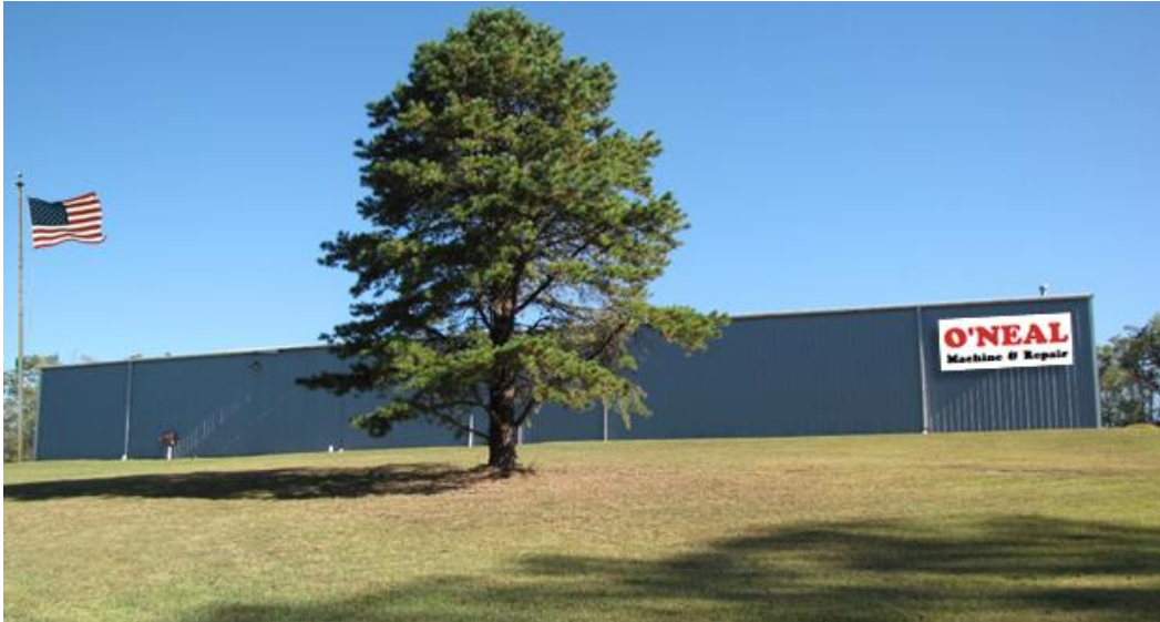
O'Neal Machine & Repair 22,000 Sq. Ft. Building
