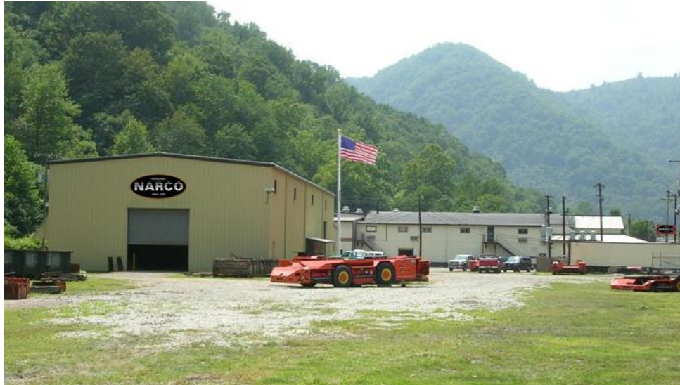
View of NARCO Plant in Smithers, WV
