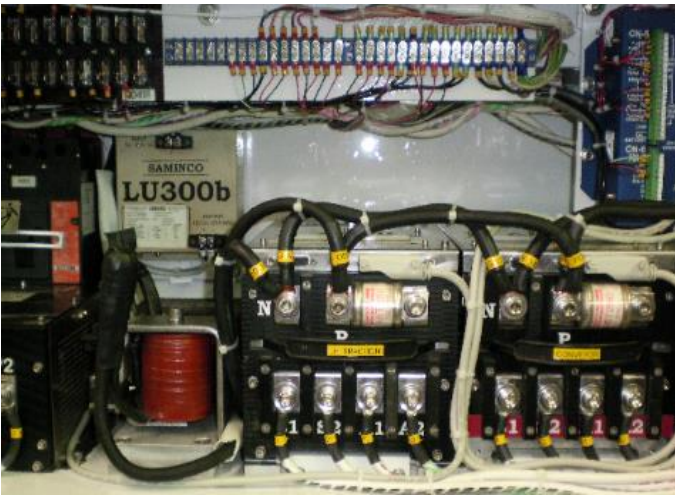
Reconditioning of Mine Electrical Enclosures
